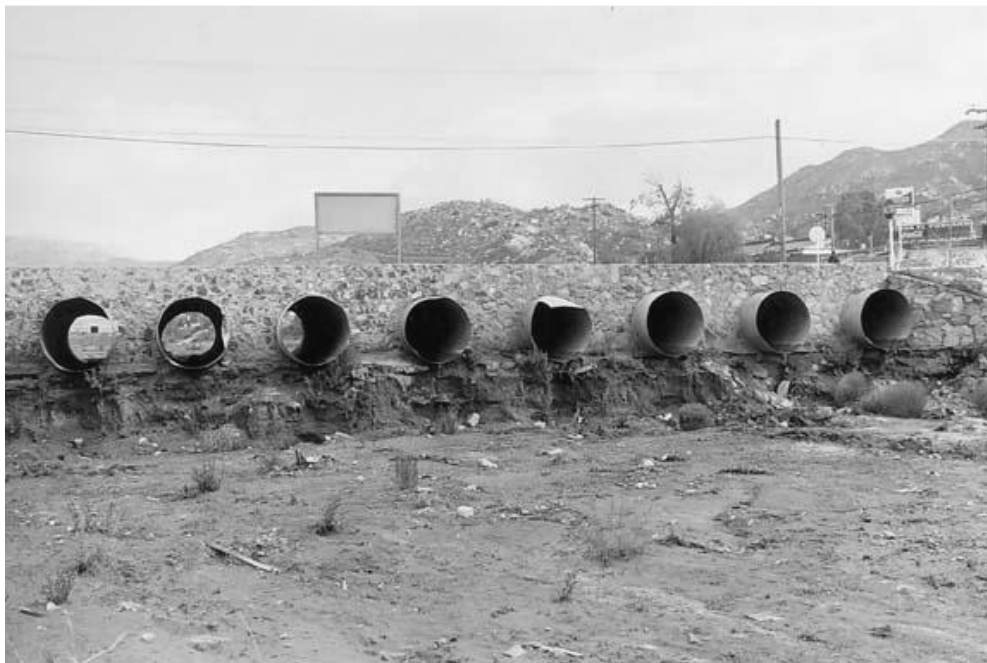
Figure 15. Tecate Creek near El Descanso, Tecate, showing extent of channel degradation
