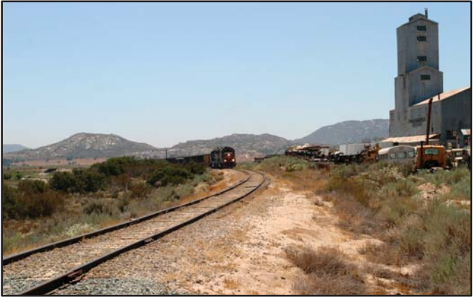
Railroad is again moving freight through the watershed between Tijuana and the Imperial Valley. El ferrocarril de nuevo transporta carga a través de la cuenca entre Tijuana y el Valle Imperial.
